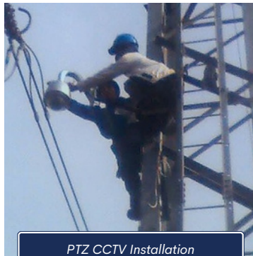
PTZ CCTV Installation
